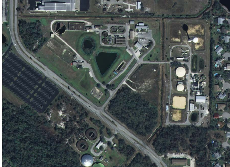
Photo of the Troutman Treatment Facility located at 1105 Troutman Blvd
